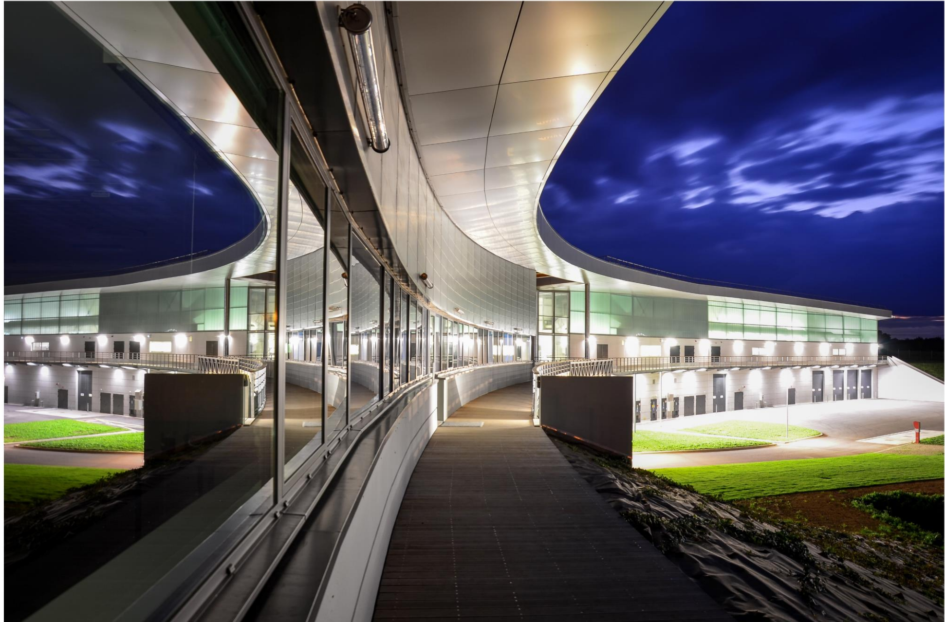
STATION D'EPURATION DE CHARTRES (28)
