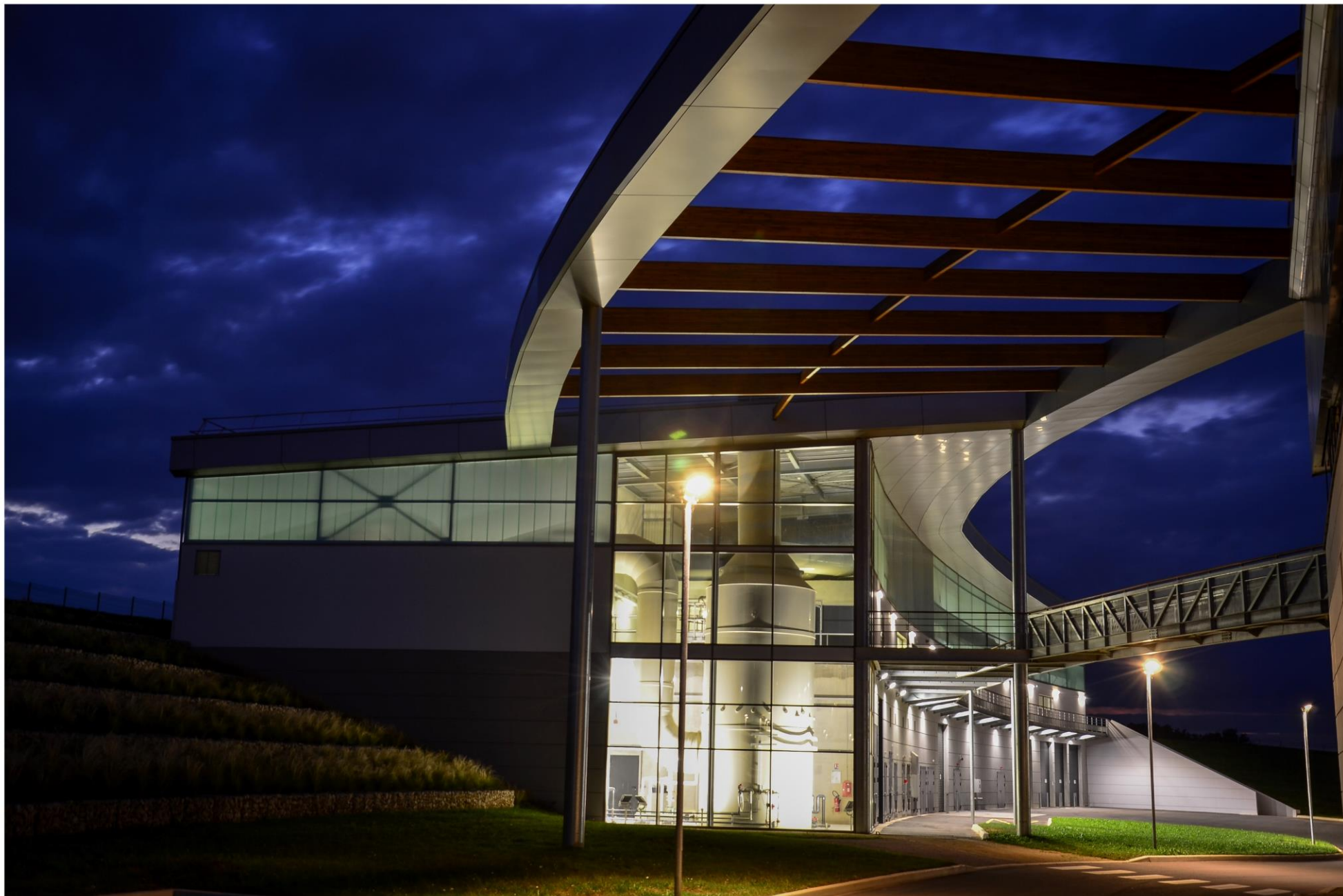
STATION D'EPURATION DE CHARTRES (28)
