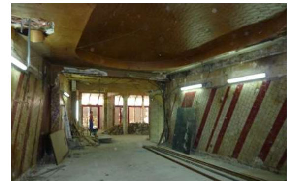
PHOTOGRAPHIES APRES DEMOLITION
