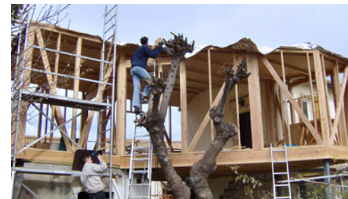
Extension ossature bois
