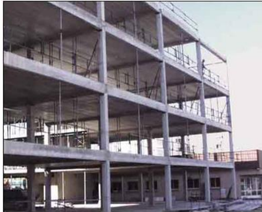
Ossatures Poteaux-Poutres
