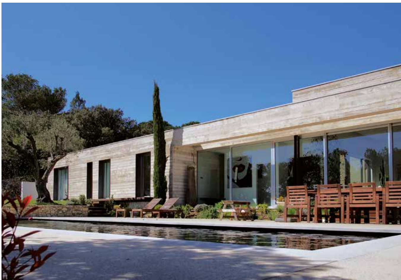
Maison individuelle, Nîmes (30), 2013, Anthony Pascual arch. © Pascual Architecture
